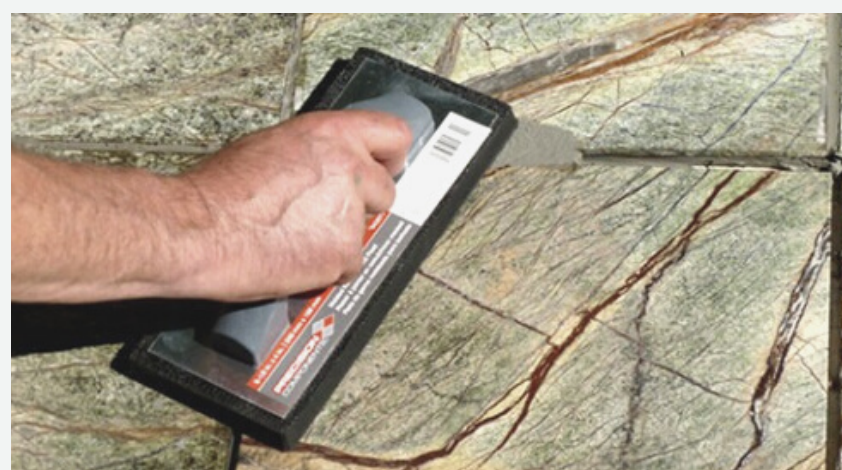
Posa in opera
